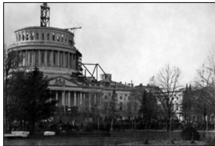
Capitol dome under construction during inauguration of President Lincoln
